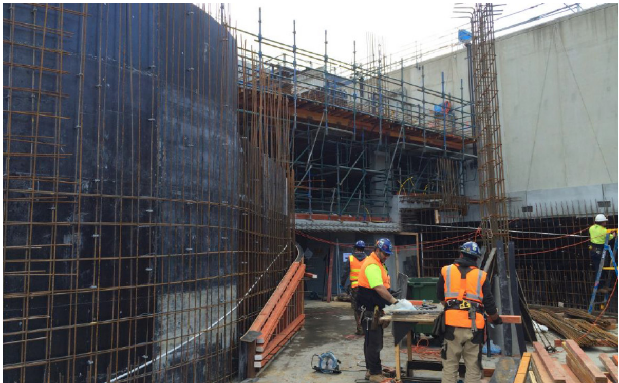
Forming of Car Park Ramp Walls
