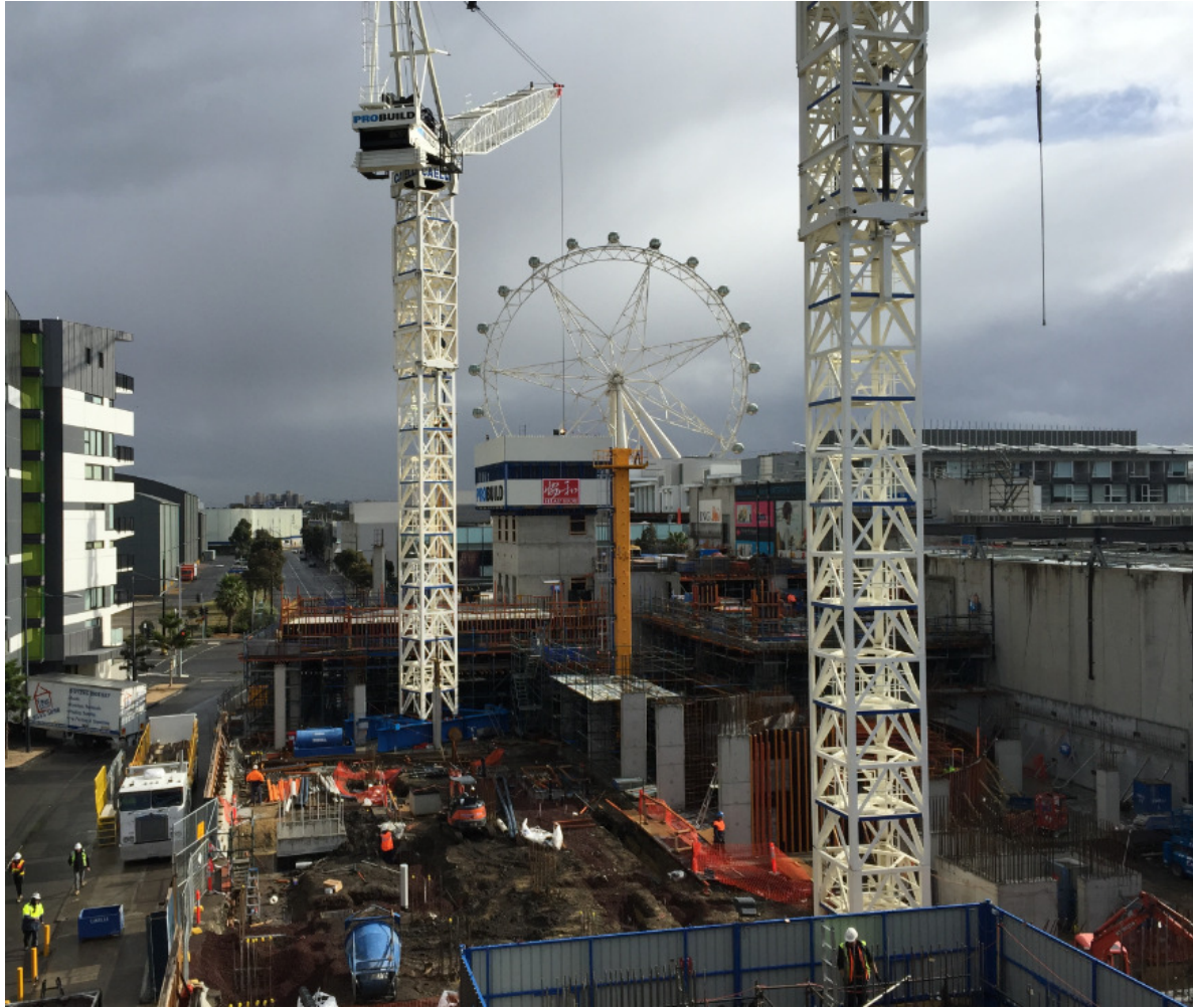
Site Overview of the Hotel Structure
